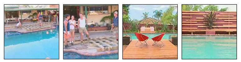
**Seating:** A rectangular frame of 90x45mm treated timber was contructed and 450mm centres noggins were fixed. Framework was then dynabolted between brickwork of garden beds. At this stage, decking timber was used and nailed directly to the frame for seating.
